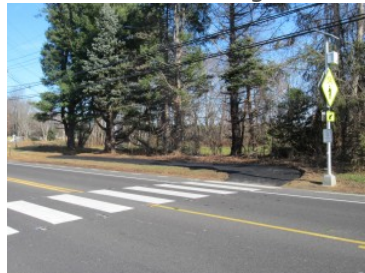
Local Road with Flashing Beacon
